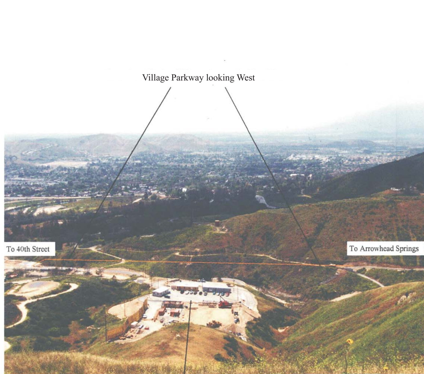
Metropolitan Water District Tunnel Site
