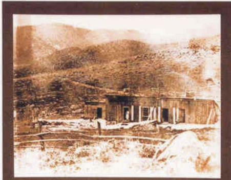
The first building at Arrowhead Springs was Dr. Smith's "Hot Springs Inlet," built in 1864. It was built over the spring which was used for medicinal purposes until 1902 (just a year after the town was founded).
